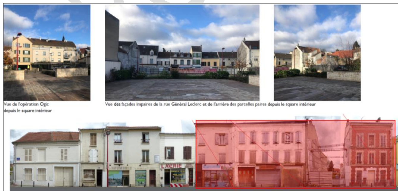
FIGURE 5 ILOT LECLERC PAIR, REPORTAGE PHOTOGRAPHIQUE AVANT/ APRES DEMOLITION
